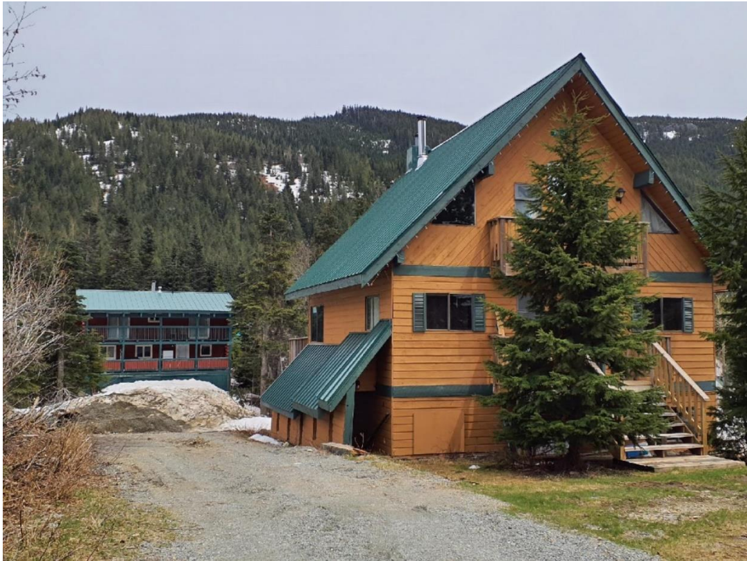
Figure 9. Older home with non-compliant lean-to, wood siding, and conifer vegetation within 10 metres of the home.
