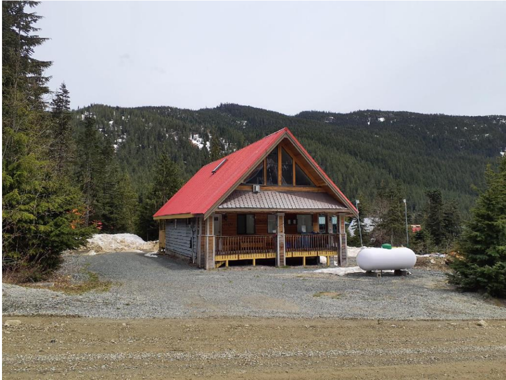
Figure 7. Home with defensible space, but combustible open deck and wooden sidings.
